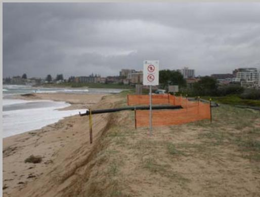
**Photo 6** - 8<sup>th</sup> February 2008 – severely eroded beach profile with pipeline discharge prepared for beach nourishment activities
